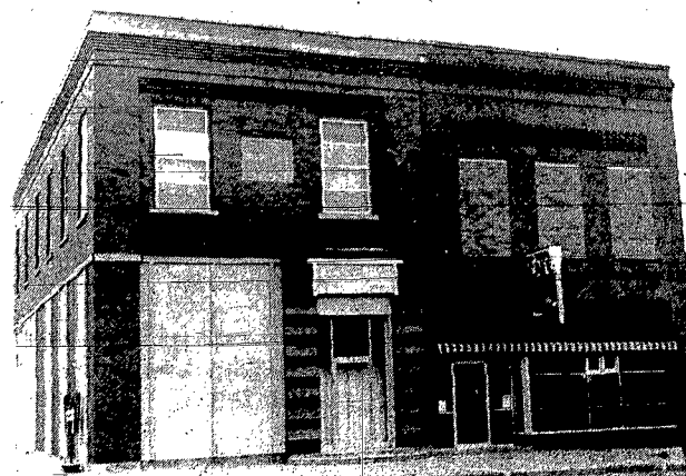
THESE ARE the buildings in Wakefield for which the Educational Service Unit 1 board of directors paid $55,000. A minimum of $17,000 will be required for renovation before the facility is ready for occupation in July. Potential problems involving the use of the three-story buildings by handicapped persons are yet to be resolved.
